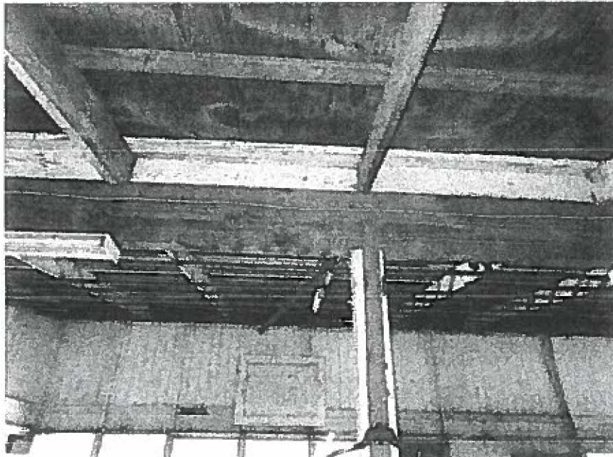
Photo 9 – Typical beam to intermediate post connection
